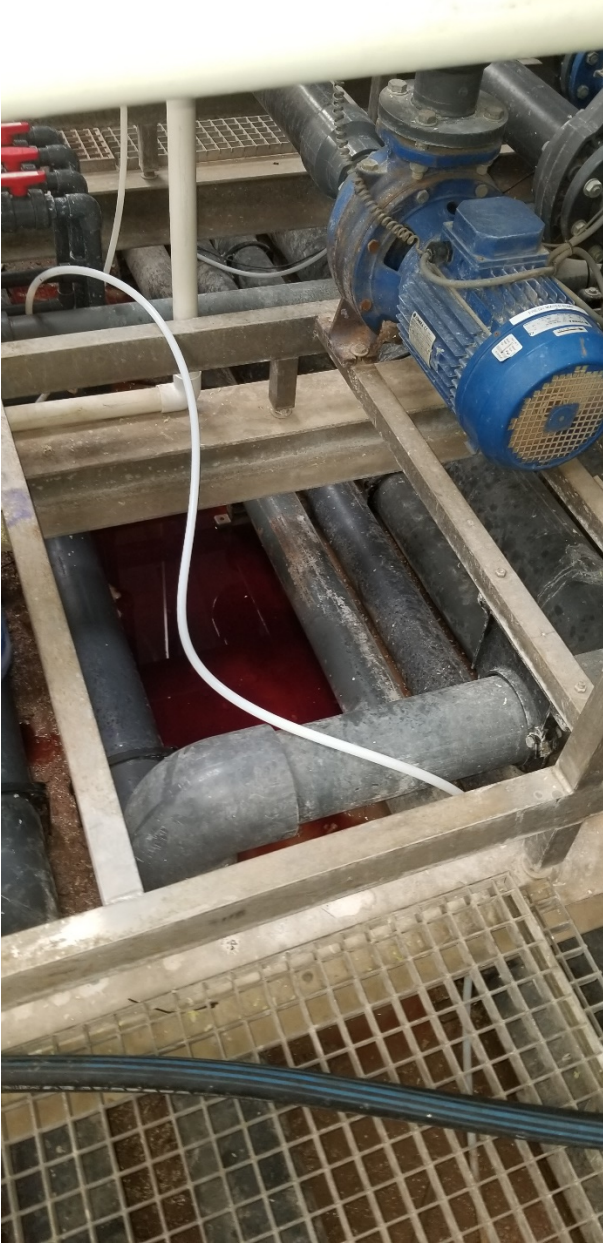
Photo 9: Inside the fertilizer warehouse, ADEQ observed standing red liquid within the secondary containment for the irrigation system's pump. The red color was similar red liquid in a tub labelled "Fertilizer." ADEQ asked for a copy of the SDS for the fertilizer with red color.
