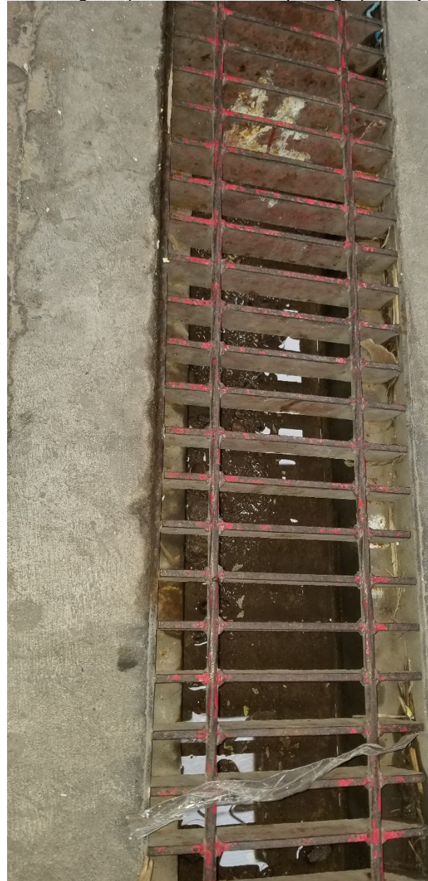
Photo 10: Copperstate representatives explained that the floors within the fertilizer warehouse are cleaned using a hose and all wastewater is directed toward the surrounding sumps.
