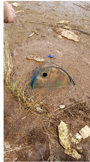
Photo 8: The top of the drum was finally exposed. The words "Waste Diesel" are painted in red on the top of the drum. The drum was open.
